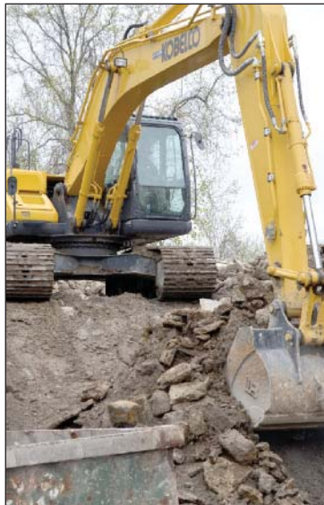
Metro Green's Kobelco SK210 LC-9 increased the company's production and efficiency.
